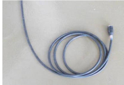
Connection cabinet and the power distribution cabinet
